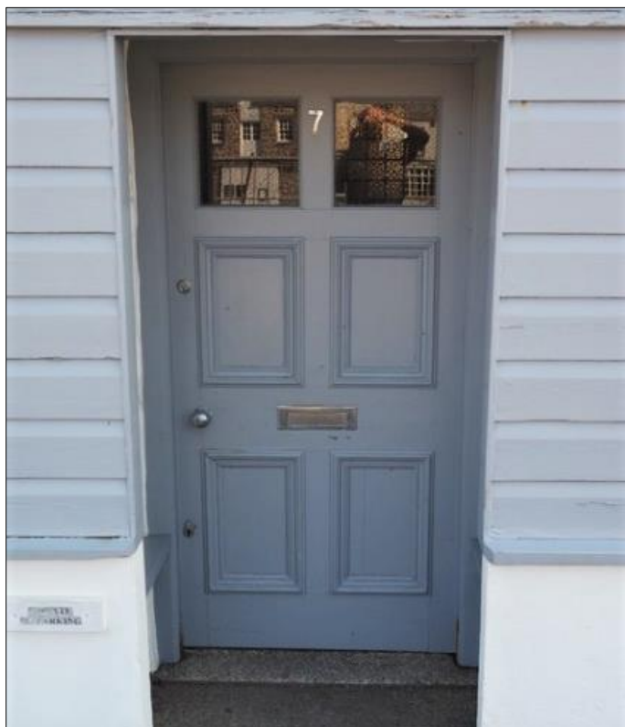
Fielded panelled front door on Quay Road.
