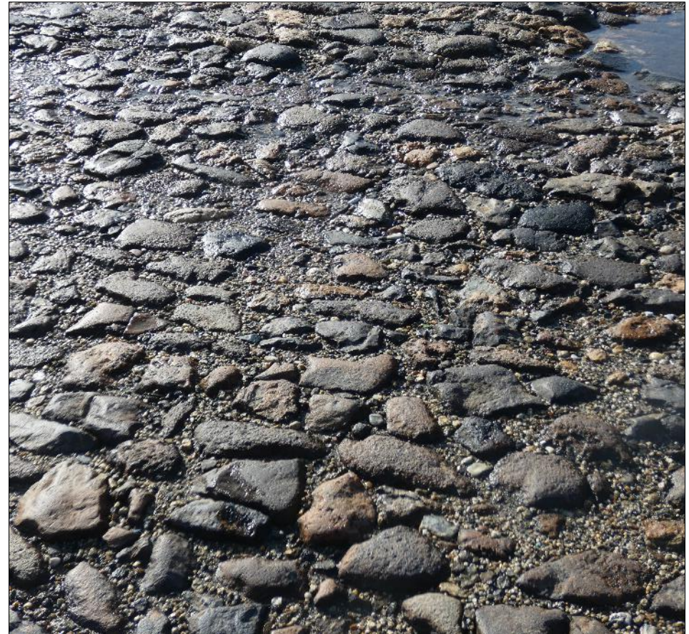
The distinctive surfacing of the former ore floor now used as the Rashleigh Arms car park.
