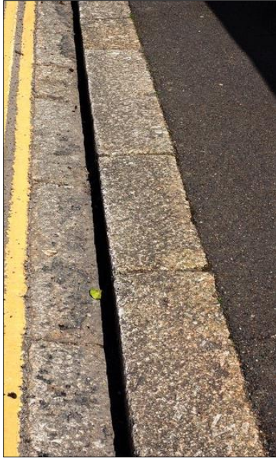
Left: wide granite kerbs and gutters. Right: narrow, roughly dressed moorstone kerbs.
