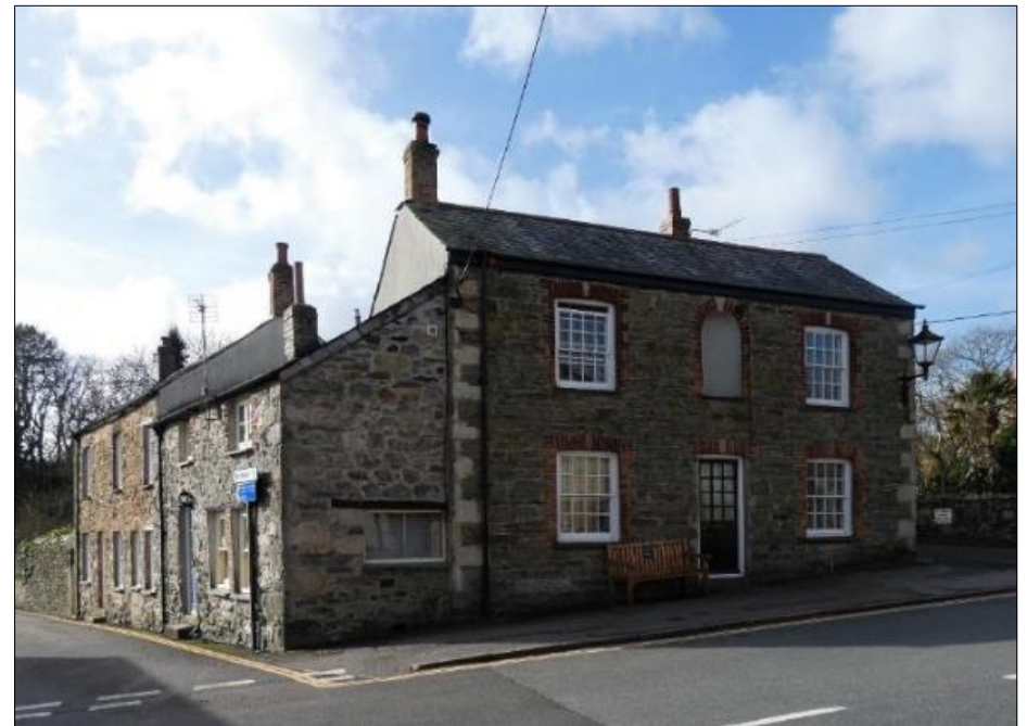
Killas, moorstone and brick in a group of houses on the corner of Charlestown Road and Duporth Road, a mix typical of many of the nineteenth-century buildings in Charlestown.
