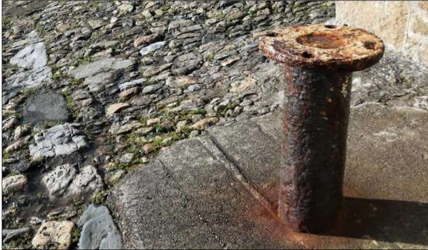
Part of a rising main from a mining or china-clay working reused as a bollard.
