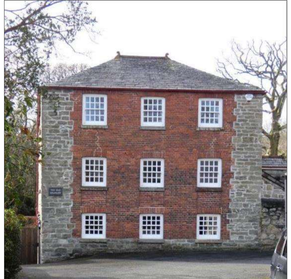
The striking red brick and granite east-facing elevation, eight-over-eight sash windows and hipped roof mark out the granary in the former farm complex on the west side of Charlestown Road as a building of some status.
