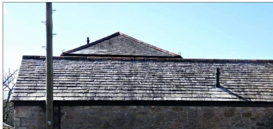
A scantle slate roof in a prominent position alongside Charlestown Road.
