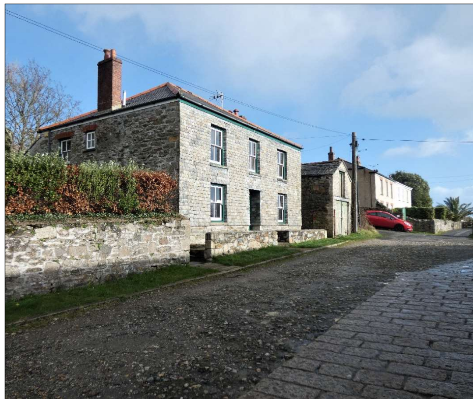
Distinctive dressed granite setts and stone metalled surfacing in Quay Road.
