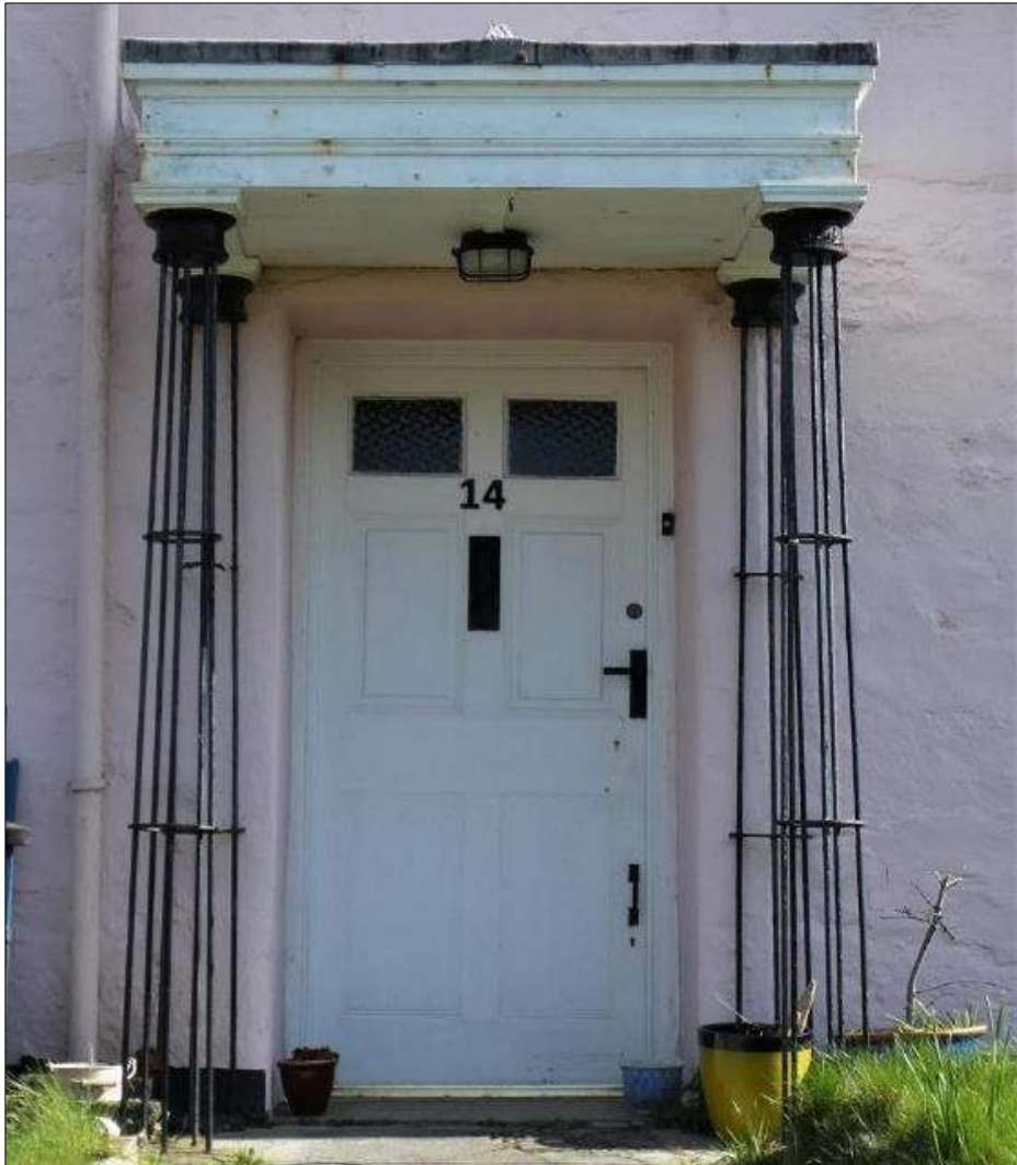
Wrought-iron columns supporting porch canopies are a distinctive element on several Charlestown houses and were probably manufactured in the village.
