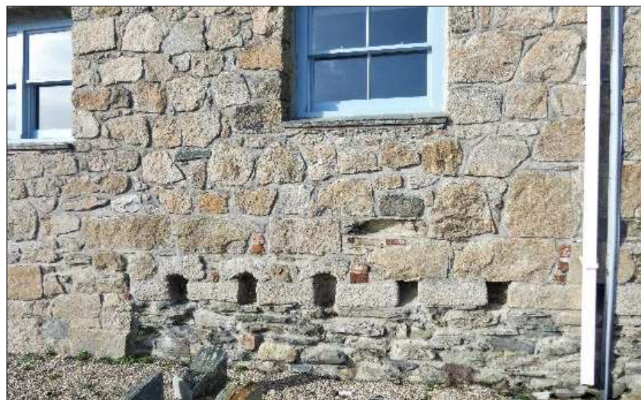
Surviving press pole sockets in the wall of the former pilchard cellar at 1 Quay Road (Salamander), now converted to holiday accommodation. The original building pre-dated the development of Charlestown.
