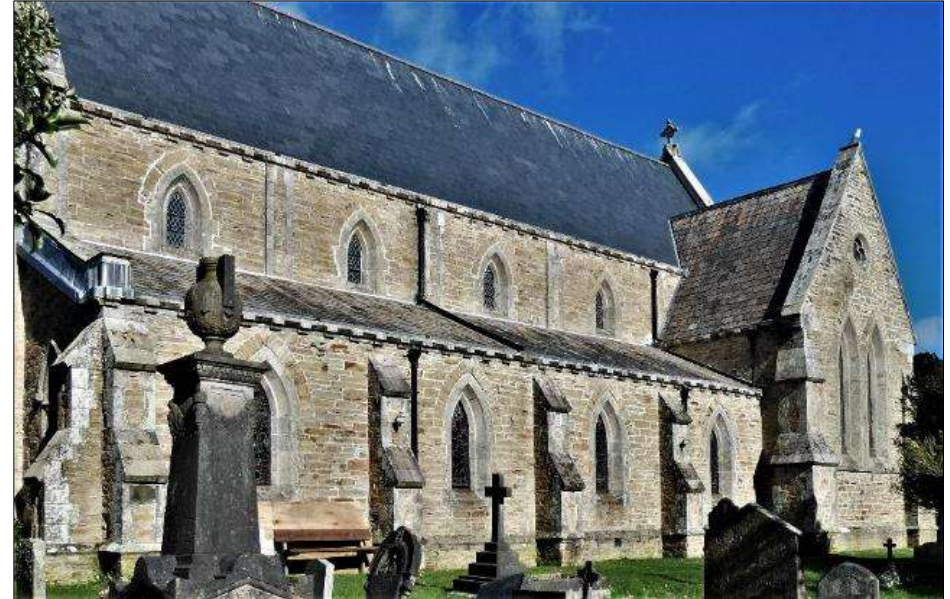
Semi-coursed dressed killas with granite dressings used for the main body of St Paul's church.
