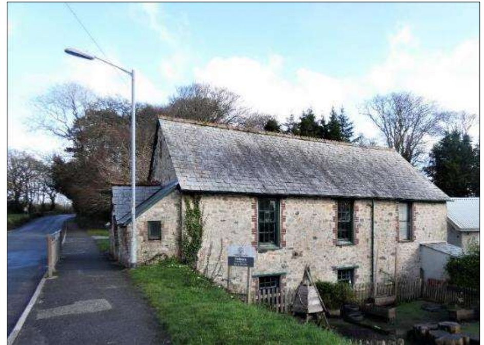
Killas stonework and brick detailing on the former Church of England Sunday School, located on the edge of the churchyard on Church Road. The utilitarian form of the street lighting is inappropriate to the quality of the historic environment and green setting in this area.
