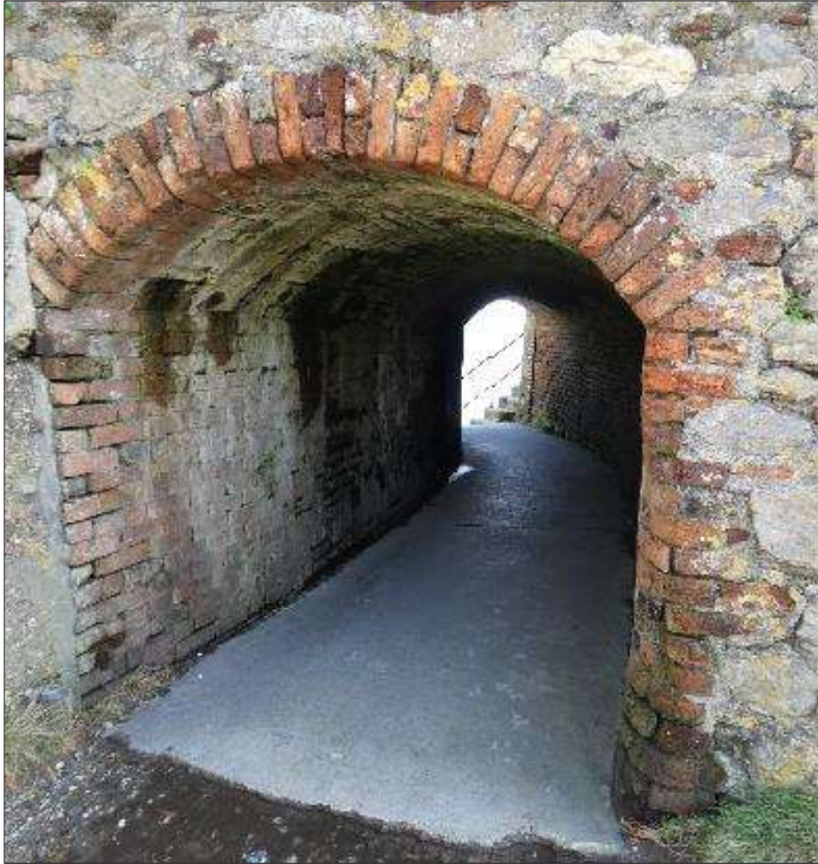
The brick-lined tunnel linking the eastern side of the inner harbour to a point above the beach.
