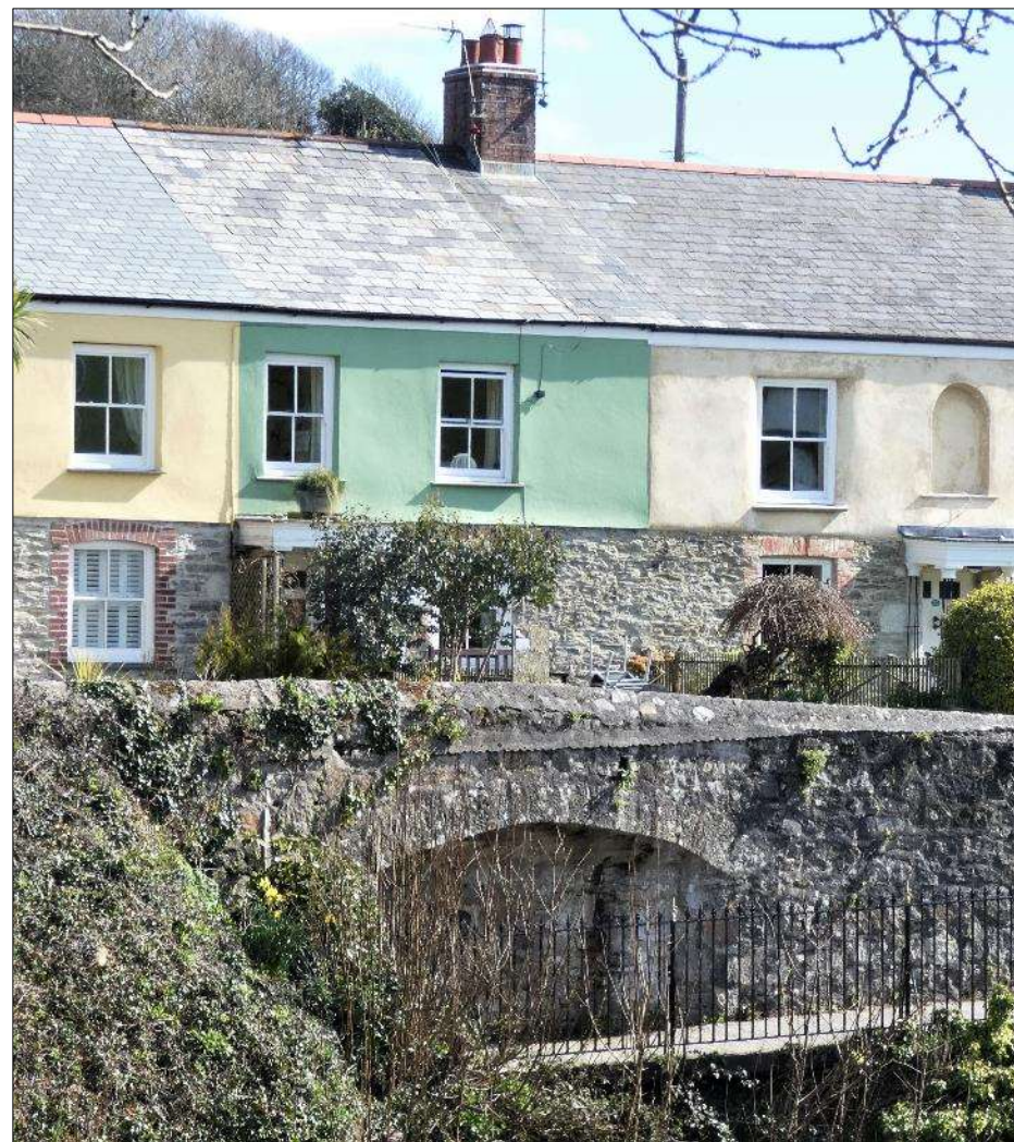
The portal to the tunnel under Quay Road which formerly carried a tramway from the Lovering clay dry to the harbour, a unique feature of Charlestown's history as a china clay port.
