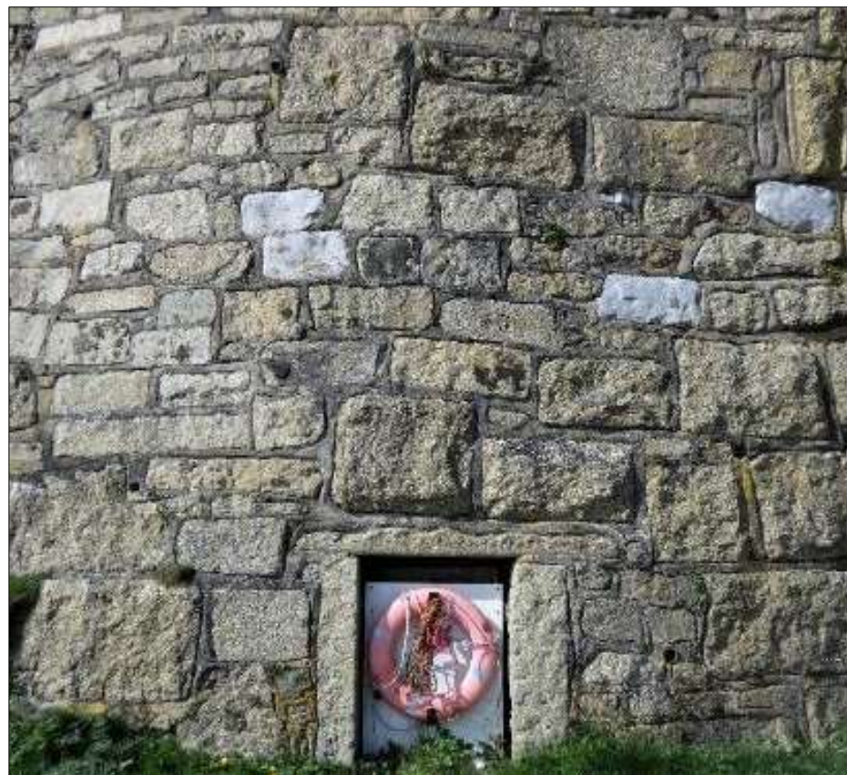
Massive moorstone (granite) blocks face the retaining wall to the west of the outer harbour.
