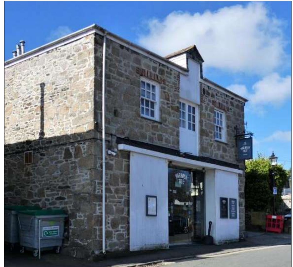
Former use as a warehouse can be read in the surviving large ground floor opening and gable dormer which would originally have housed a hoist.
