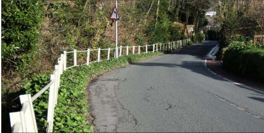
Railings along Duporth Road; the uprights are lengths of former tramway track. The earthwork embankment to the left encloses the Lower Pond.
