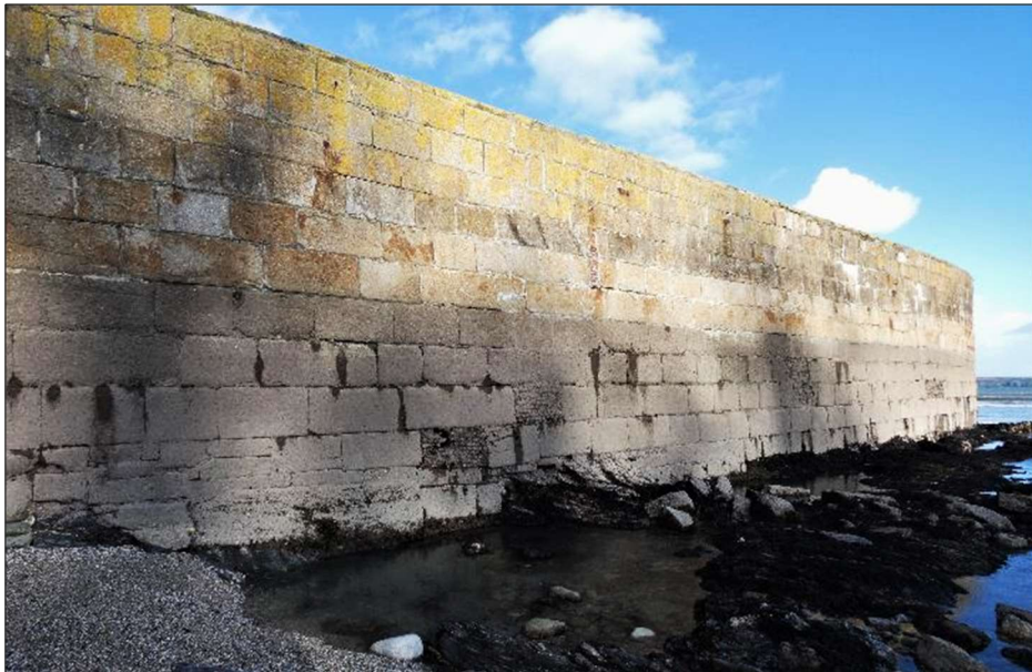
Massive moorstone blocks and old repairs in brick on the seaward side of the Grade II* Listed outer harbour wall.
