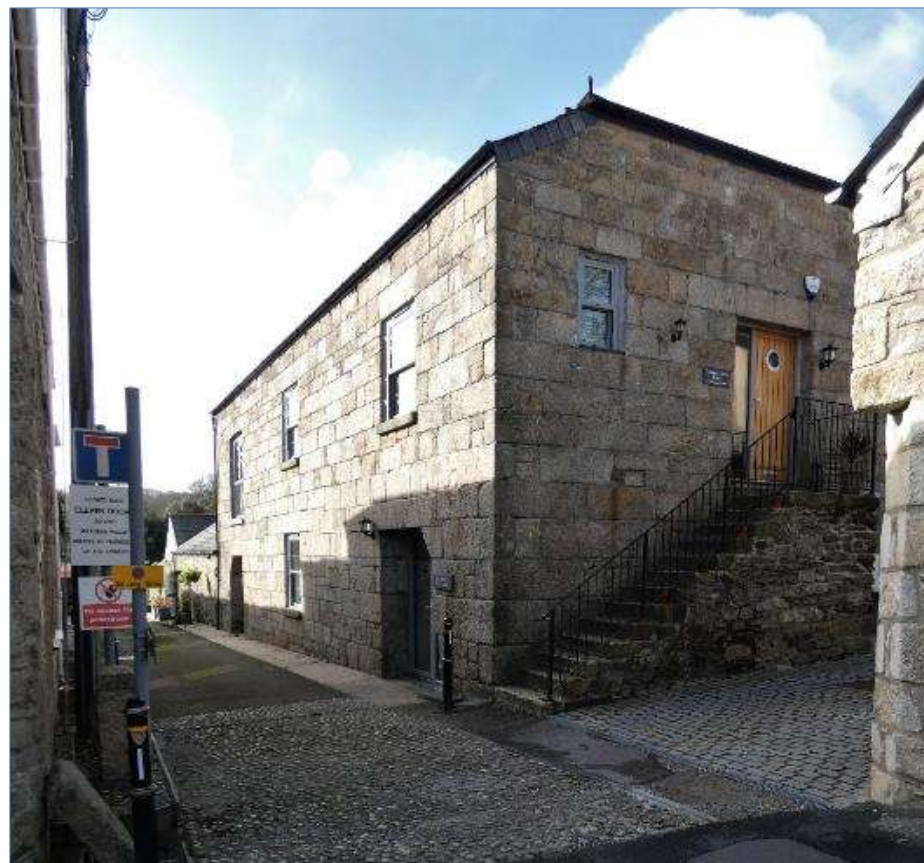
The former water-powered threshing barn, later used as a china stone mill, on the north side of Eleven Doors. It is constructed from finely dressed moorstone granite.
